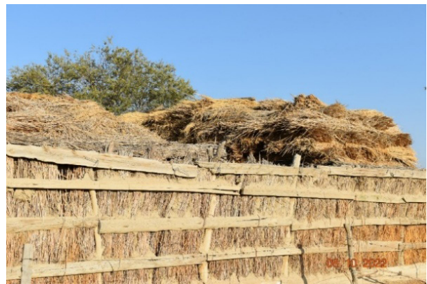
Figure 4 – An example of the use of reed as a building material
